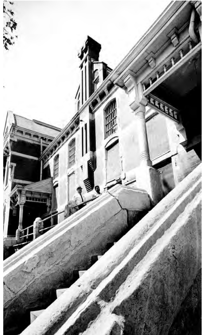
1963 Shawnee County Jail "poor condition" Topeka State Journal - Staff
