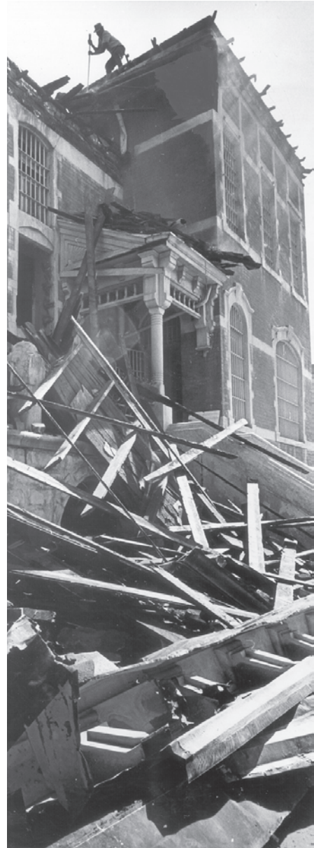
May 1966 Old County Jail being demolished. Topeka State Journal – Jack Kenward
