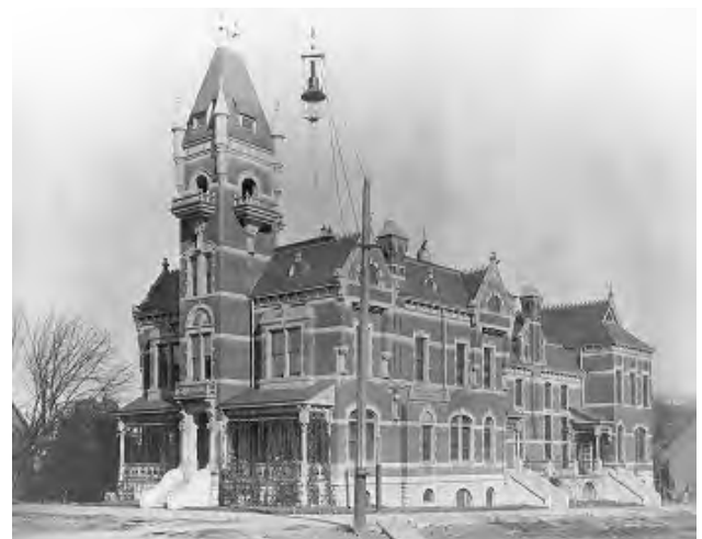
1886 Shawnee County Jail & Sheriff's Residence. Andrew Fuller is believed to be the first Sheriff to live in the residence.
