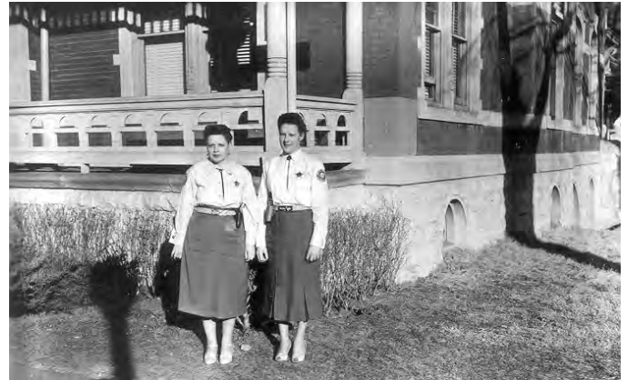
1953 Office Deputies Pearl (Lydic) Engstrom & Pauline Paige in front of Sheriff's residence and Jail at 5 th & Van Buren
